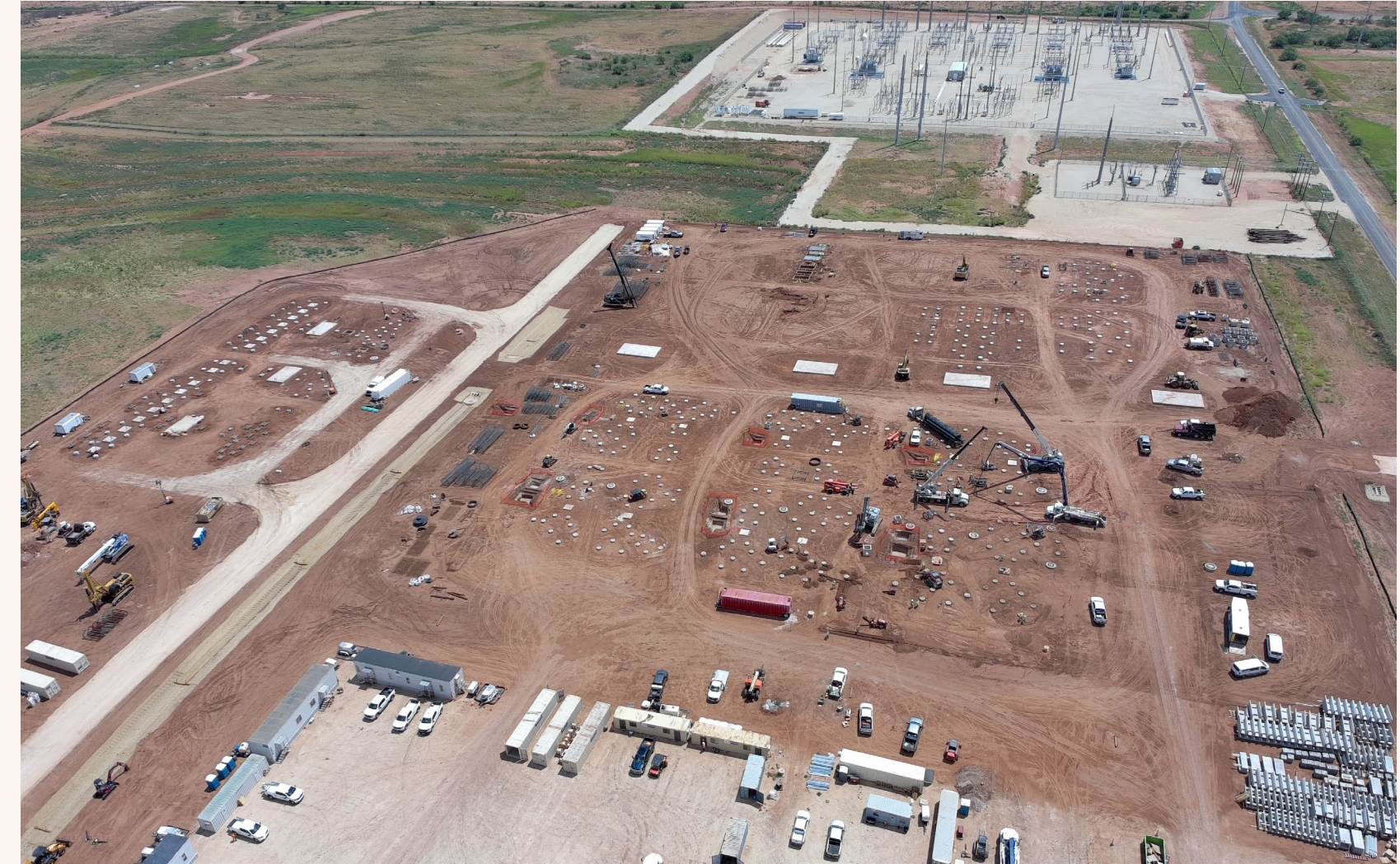
Substation construction progress at Sweetwater 1 (August 2025)
