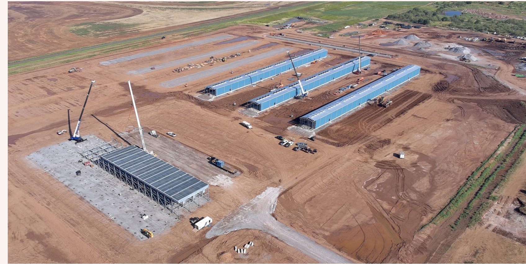
Construction progress at Horizon 1 & 2
