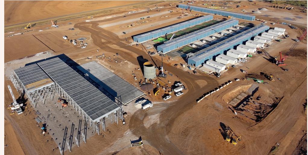
Horizon 1 construction progress (October 2025)
