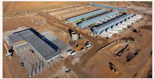
Horizon 1 construction progress (October 2025)
